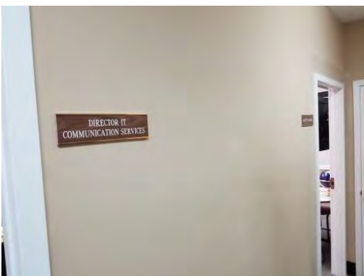
Item: 7 Signage does not have raised letters and braille, typ.
