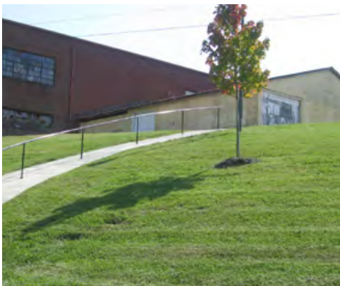
This park ramp needs to be redesigned to meet ADA requirements.
