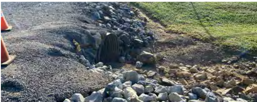
The placement of additional rip rap would prevent further erosion in this location and several others on site.
